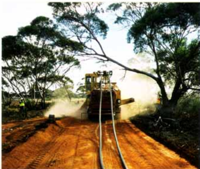
■ Construction of Murraylink HVDC Light® (Australia).
